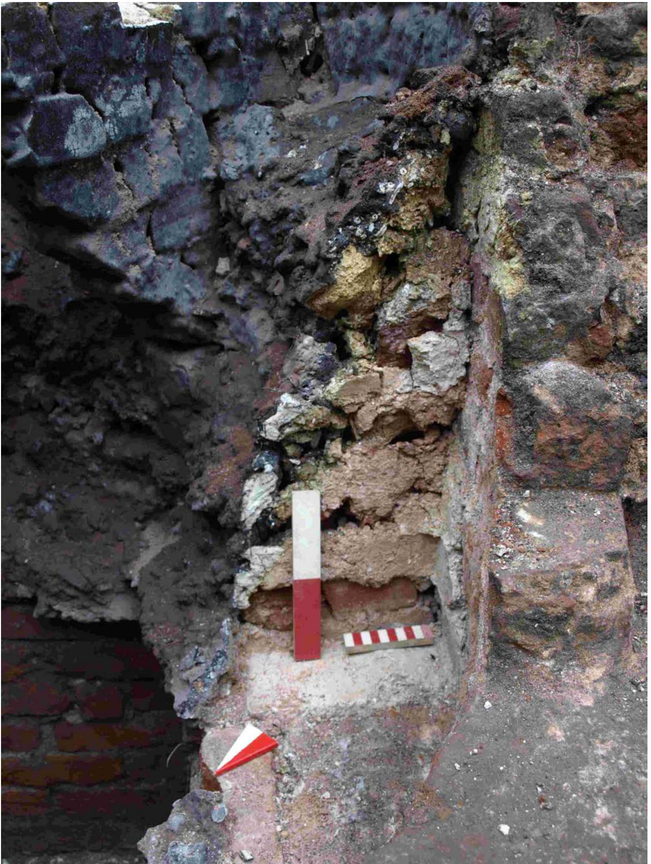
Plate 12: rubble infill between radial supports 216 and 215 (216 removed)
